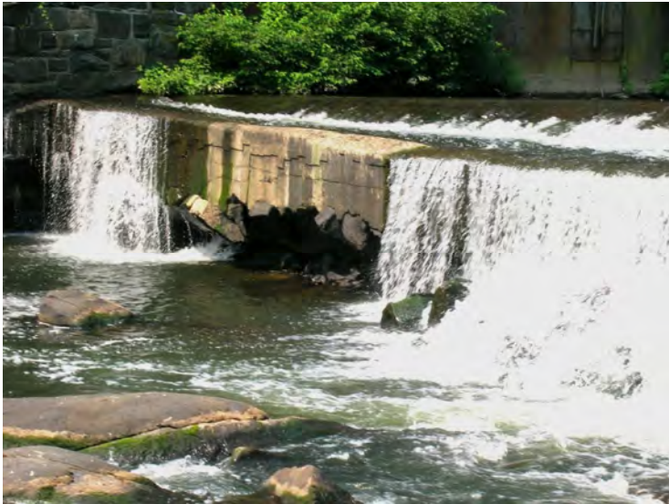
Bancroft Dam 4, damaged in center of dam
