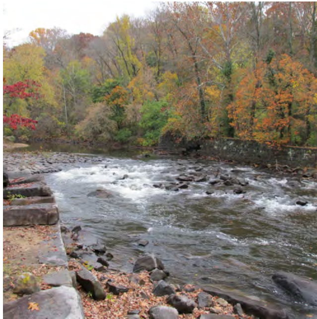
Augustine Dam 3, breached
