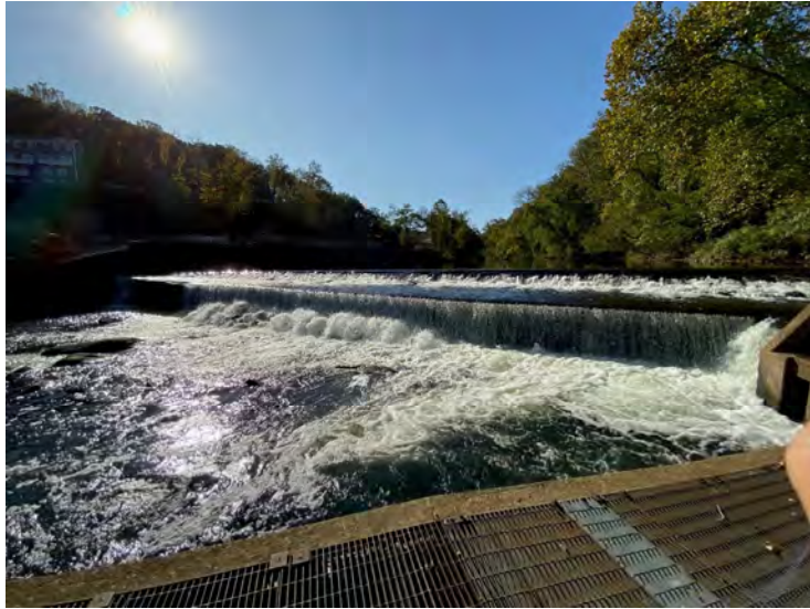
Bancroft Dam 4, damaged in center of dam
