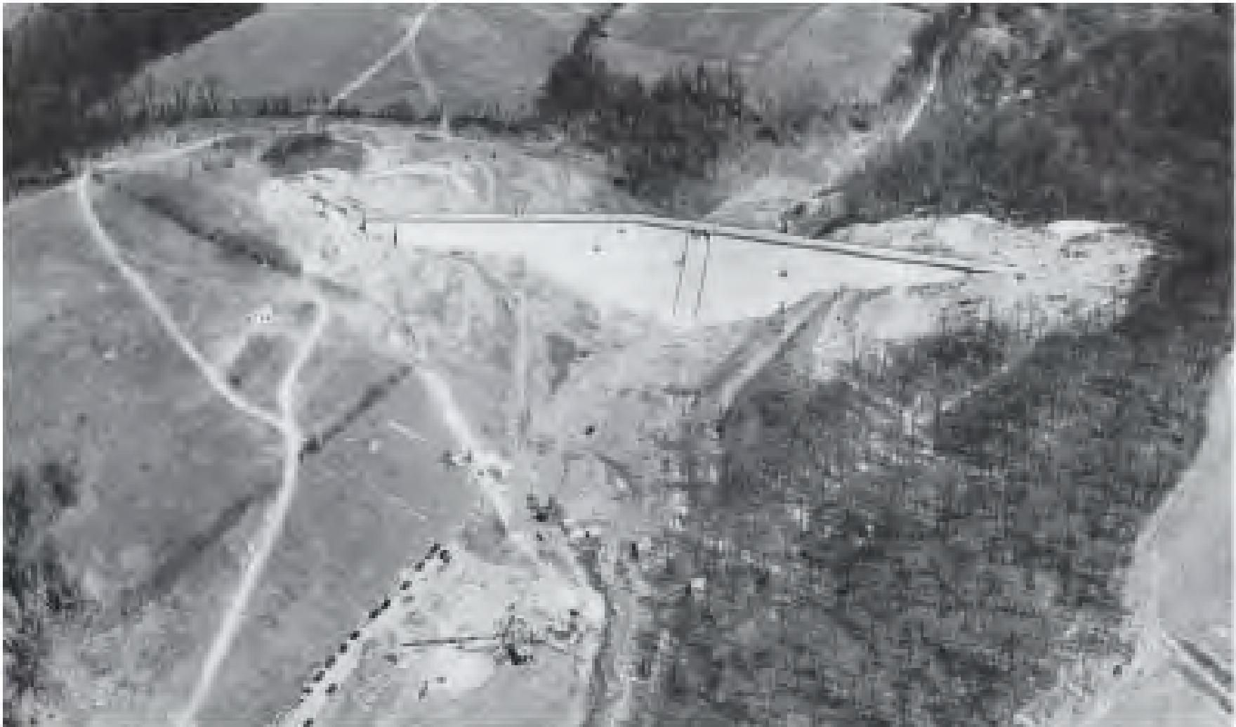
Hoopes Reservoir under construction, 1931.
