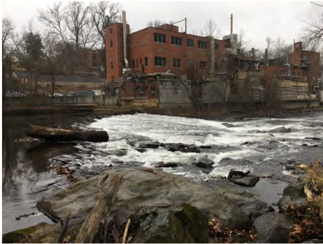
DuPont Dam 6, breached
