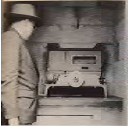
FLOW GAUGE installed on lower Brandywine measures and records volume of water going down the stream. These data help in compiling topsoil loss.
