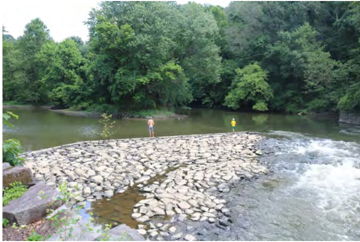
Augustine Dam 3, breached
