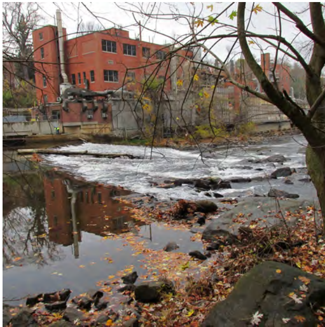
DuPont Dam 6, breached
